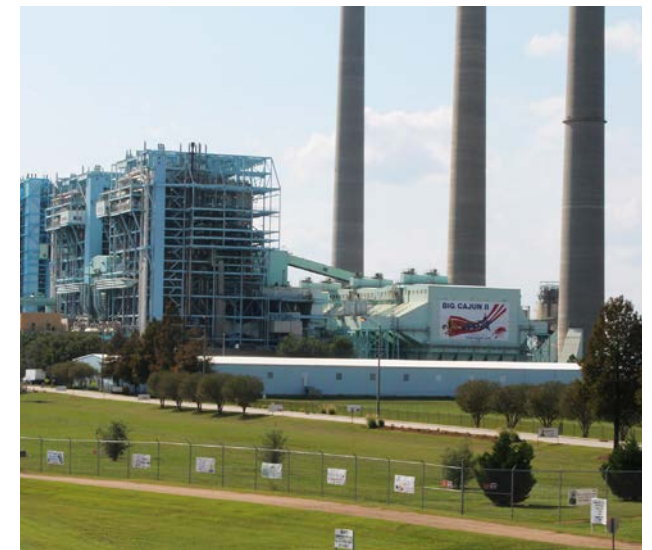
Big Cajun II Generating Station's Unit 2 now runs on cleaner natural gas, cutting its CO 2 emissions by almost 50 percent.
