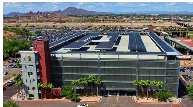
Our CHP plant at Arizona State University provides heating, cooling and electricity to the university's distribution system.
