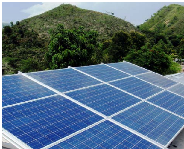
NRG helped design and install three 20-kW solar arrays in Haiti.
